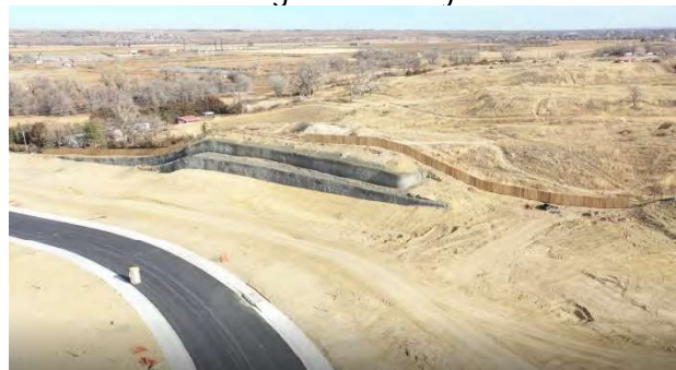
Filing 3 Retaining Walls
