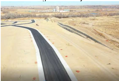
Filing 3 Retaining Walls
